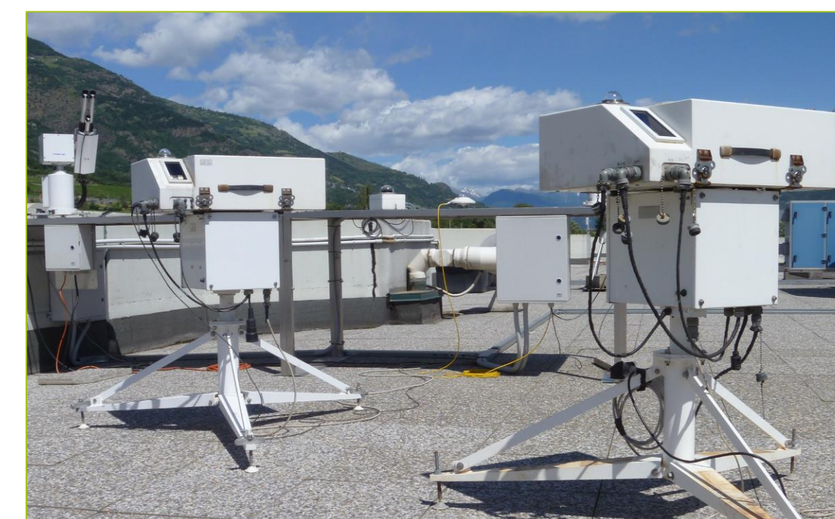
Figure 2: instrumentation at the solar observatory at ARPA.
