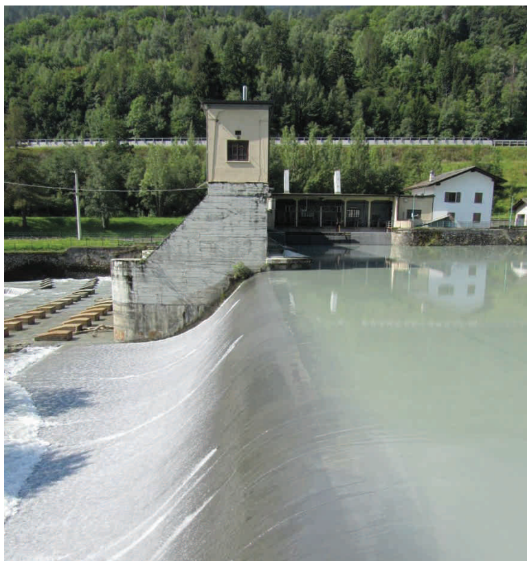
Figure 22 Hydropower facilities along the Dora Baltea river [taken from ARPA (2012)].
