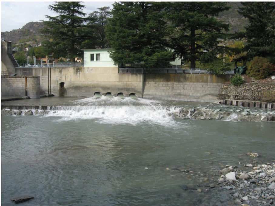
Figure 21 Hydropower facilities along the Dora Baltea river [taken from ARPA (2012)].
