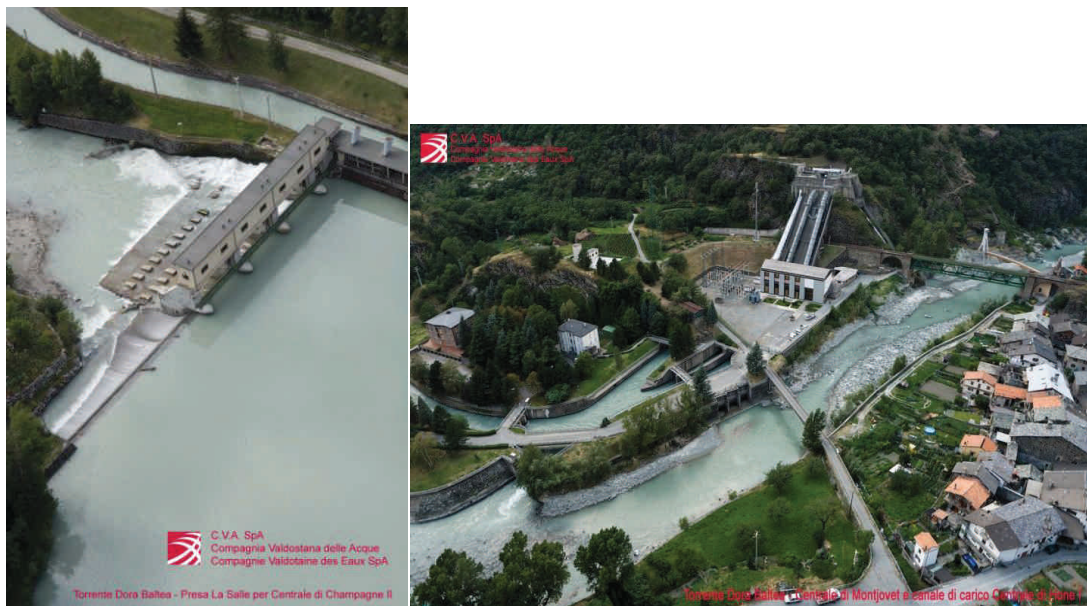
Figure 14 La Salle intake and Montjovet intakes [taken and modified Regional Energy Plan, RAVA – 2003].
