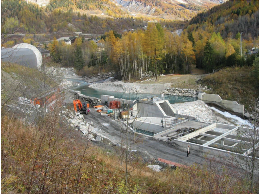
Figure 20 Hydropower plant building along the Dora Baltea river [taken from ARPA (2012)].
